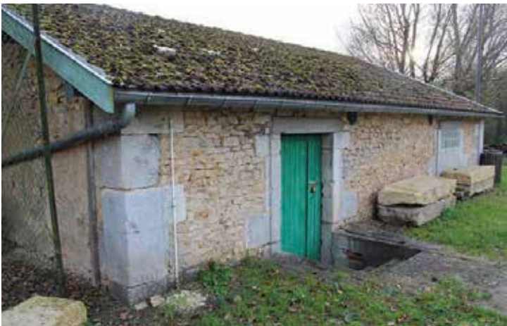
▲ The building SSgt Glen Alfter hid in after his plane went down.
