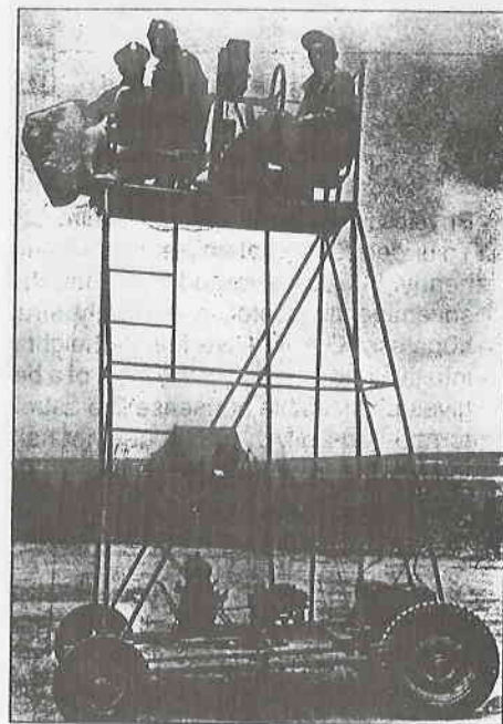
"World War II powered bombing trainer. The bombardier sighted his Norden bombsight on a powered 'crab' target. The movement of the trainer across the ground simulated the movement of the aircraft and the movement of the 'crab' target simulated the effect of wind causing the aircraft to 'crab' or drift relative to the target." [From America's Pursuit of Precision Bombing, 1910-1945 ; USAF Historical Research Agency]
